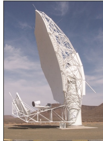
Current planning leads to Meerkat style pedestal antenna w/ feed low configuration & challenging mechanical design
